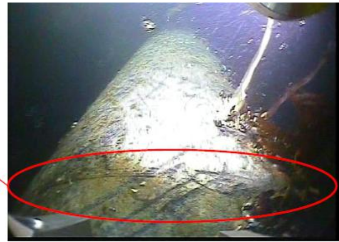
Above image is from the ROV during the inspection of Leg B2. Note the weld is clearly displayed
