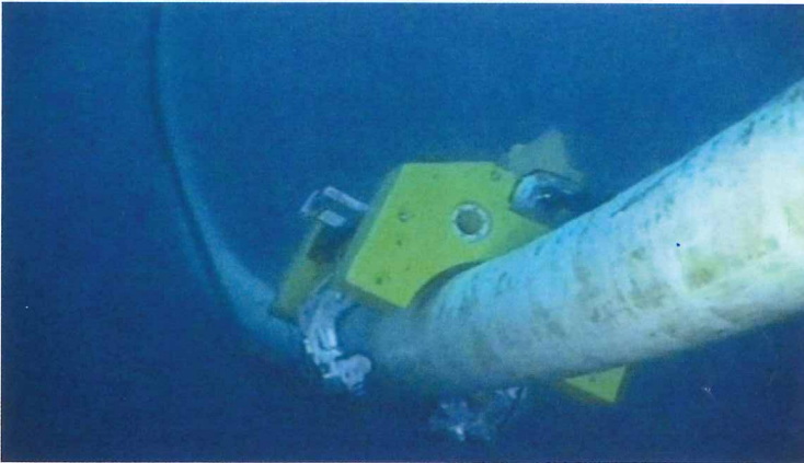
Figure 2. MEC-Hug Crawler inspecting through the sag bend of the flexible riser.
