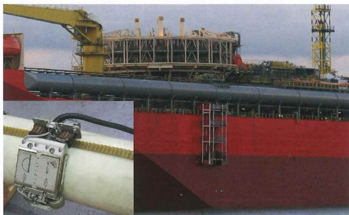
Figure 4. Flexible riser sections in the turret drag chain on the FPSO.
