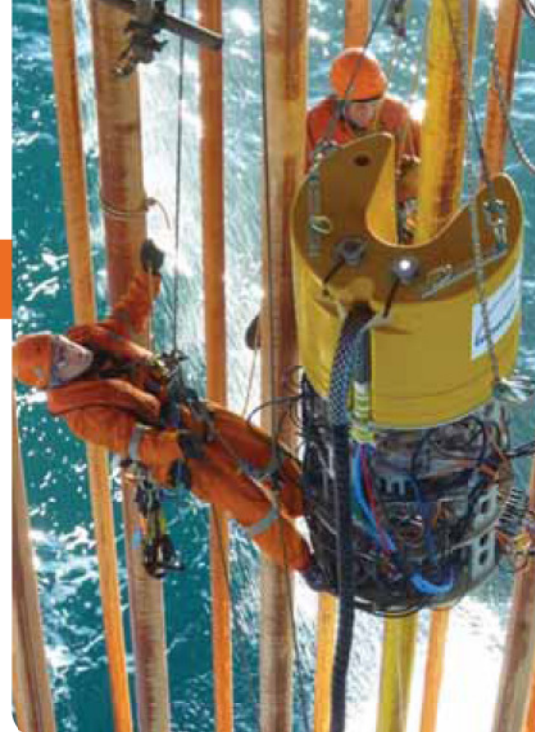
MEC-HUG riser inspection system in deployment from the installation and in operation at flexible riser in the North Sea
